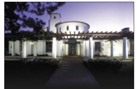
Commercial Building: Braille Institute Of America at 2031 De La Vina Street Property Owner: Braille Institute; of America; Project Architect: Brian Cearnal, Cearnal Andrulaitis Architects; General Contractor: Mark J. Melchiori, Melchiori Construction Company; Civil Engineer: Michael A. Caccese, MAC Design Associates Landscape Architect: David Niles, Landscapes by Davids Landscape Contractor: R. G. Foil, Ron Foil Landscapes Landscape Maintenance: Douglas Wasson, Plowboy Landscapes, Inc.
