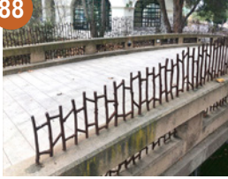
Next to the Carousel House, 223 E. Cabrillo Blvd. Untitled (Bridge) 1998 Susan Jordan Yoshimine
